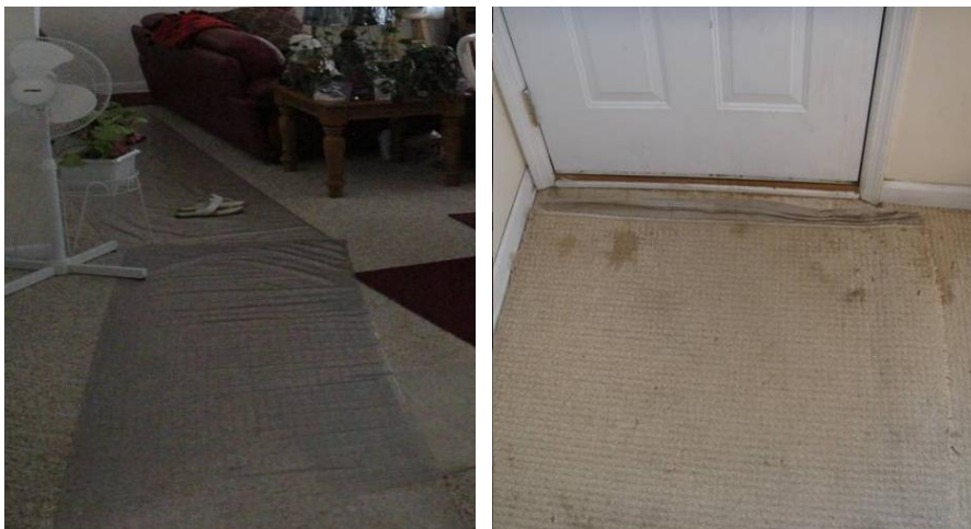
Figure 1 - 1. Examples which show clear vinyl covers or loose carpet piece over the carpeted floor
