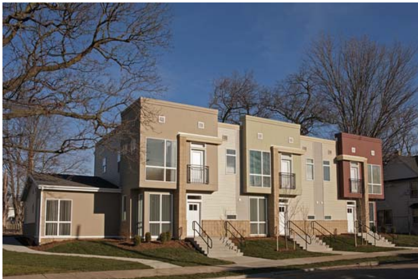
Photo Courtesy of: Orion construction, Inc
