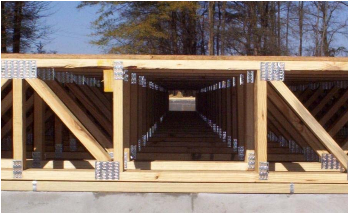
Open-Web Floor Trusses (1 point)
